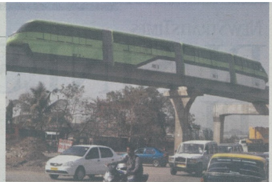
Scomi Engineering is constructing Phase Two of the RM1.85 billion Mumbai monorail project. Bernama pic
